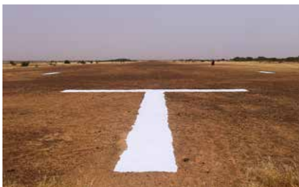
Rehabilitation of Menaka airstrip in the Gao region of northern Mali, completed through a joint WFP Mali and ACTED programme, has allowed UNHAS to continue transporting humanitarian staff. ACTED/Photolibary
