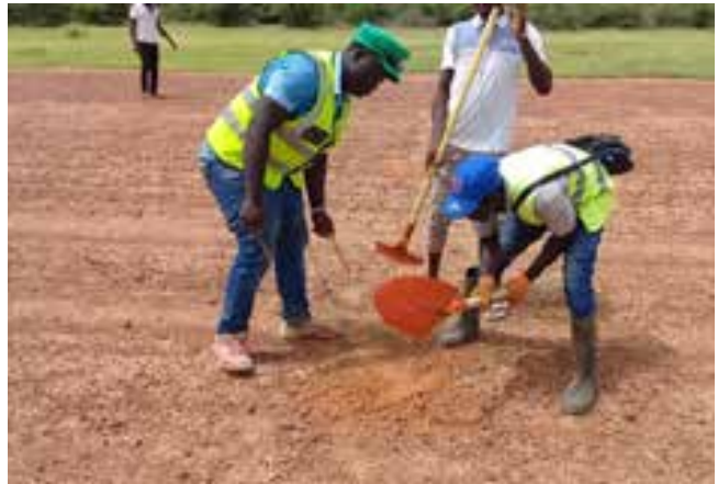
Bassikounou airstrip. Repair works: maintenance and levelling of airstrip gravel surface.
