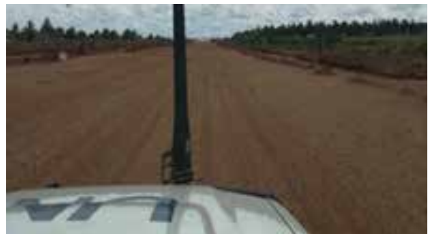
Tshikapa airstrip status in November 2019 after UNHAS repair works.
