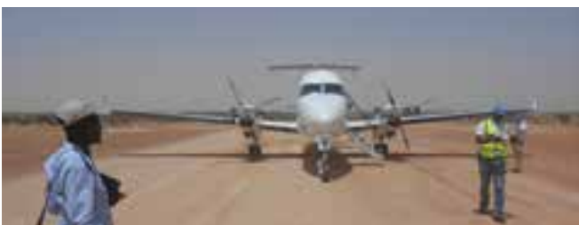
Current status of Iriba airfield (Eastern side of Chad, at the border with Sudan) after two months of repair works managed by UNHAS to allow the landing and take-off of aircraft with higher seating capacity (from 12 to 19 and 37 seats).
