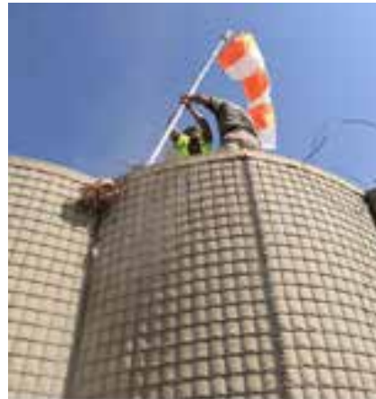
Sharana HLS (Helicopter Landing Zone), October 2019. Repair works: Windsock installation.
