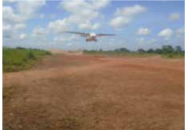
Repair works: rehabilitation of Paoua airfield.
