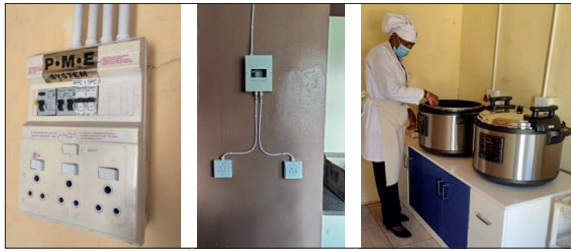
Figure 1: Adding new circuit breakers and electric sockets in the school kitchens
